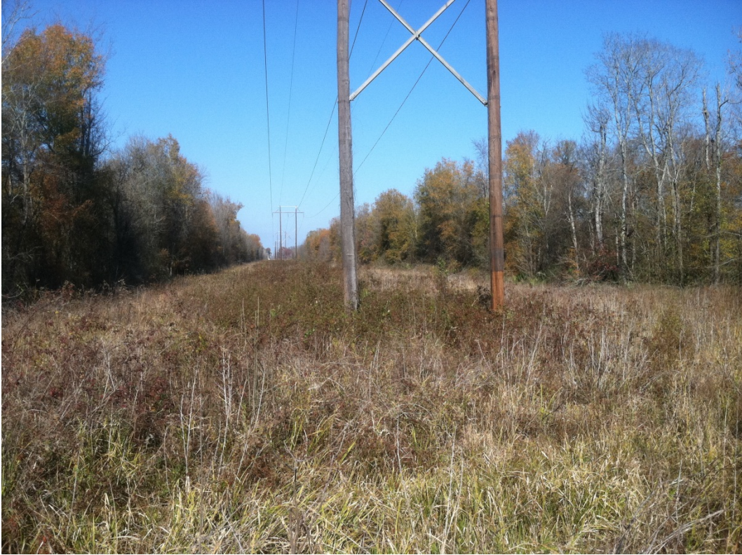
EXHIBIT 9. POWERLINE TRANSMISSION ROW.
